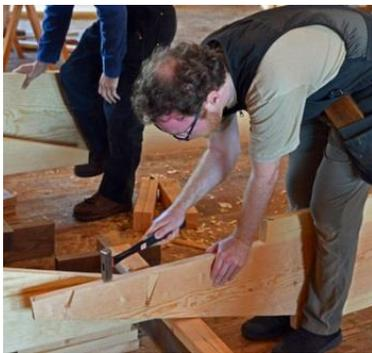
One of the methods employed to ensure tight joints is **Kigoroshi** (killing wood), in which the joint member surface is hammered to compress the wood fibers to make the joints fit better, knowing that the wood will swell back to its original dimensions once it gets wet, further tightening the joint fitup.
